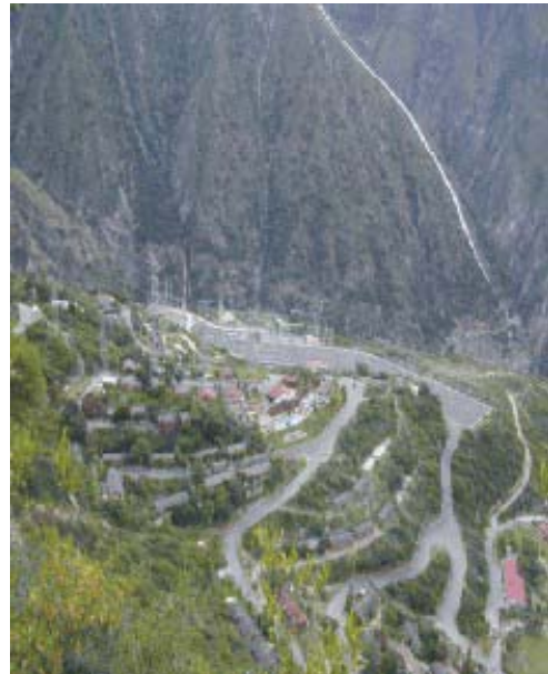
Figure 05: Partial view of the Mantaro Hydroenergetic Complex
